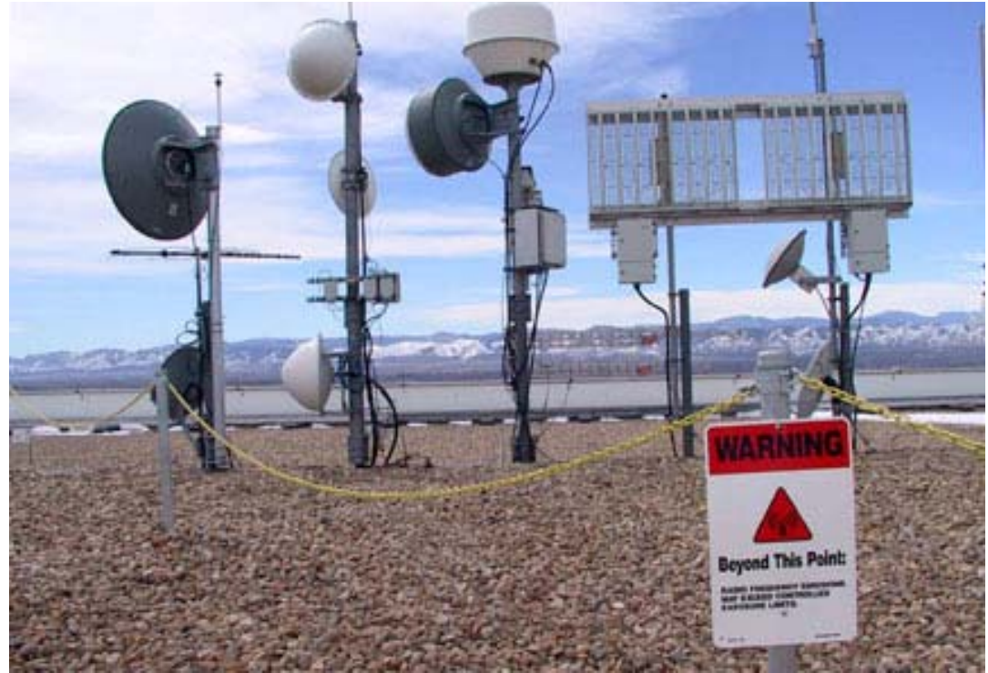
Warning Sign: "Beyond this point: Radio Frequency Exposure May Exceed Controlled Exposure Limits"
